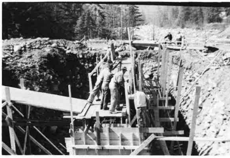
ABOVE: Working on the concrete foundation. SILVERY SLOCAN HISTORICAL SOCIETY 2020.006.011
